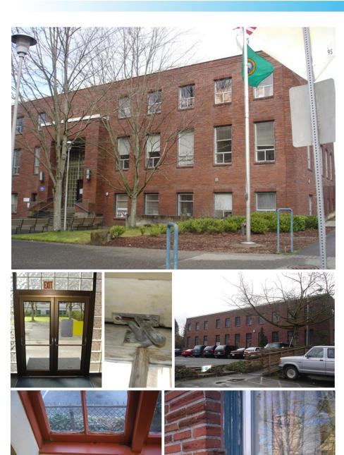
Cowlitz County requested that Merritt do an extensive study on replacing the windows and doors of the historic building. Three sides were converted to a more modern metal window and metal door system while the fourth side has maintained the original historic wood windows. This study Cowlitz helped County determine the best option to returning all four sides to the original wood windows and doors.
